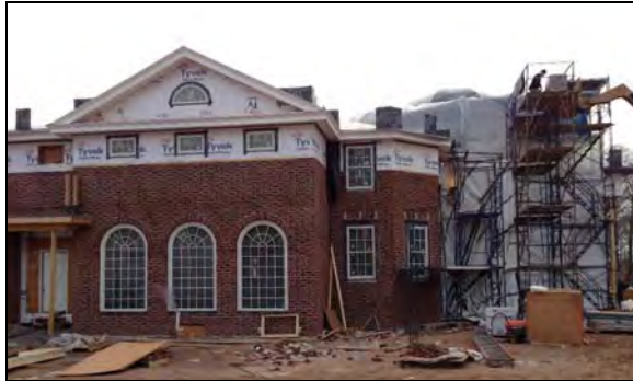
New House Under Construction
